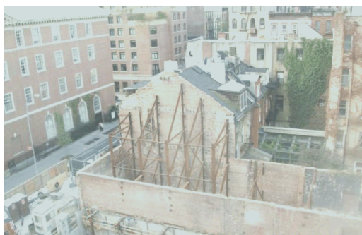
Figure 2: Shows Temporary Structural Steel Bracing
