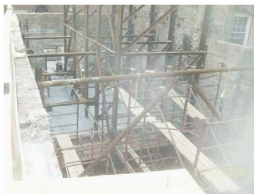
Figure 3: Shows an Up-close View of the Structural Steel Bracing
